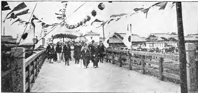
FUJINAKA BRIDGE AT OSAKA
